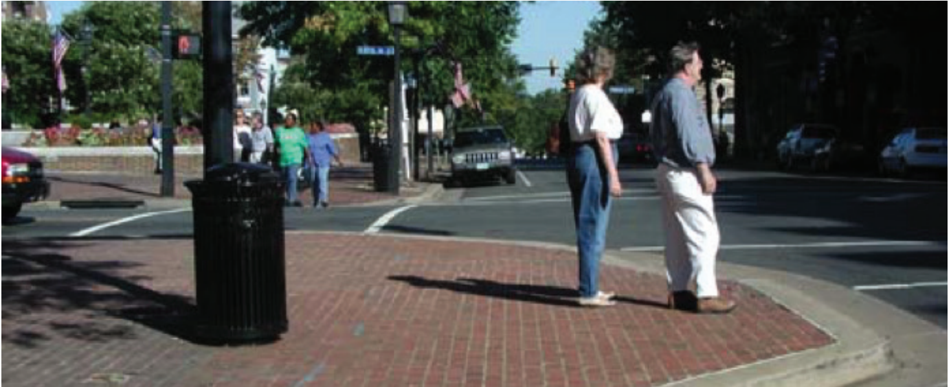
A curb extension allows pedestrians to be both closer to the other side of the street and more visible to cars.
